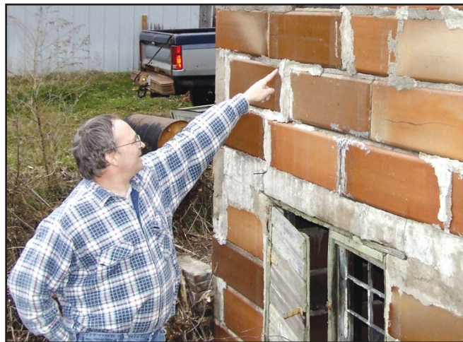
Peter Jacobs points out grout on the back wall of his sewer pipe garage. - photos by Ruth Nerhaugen
